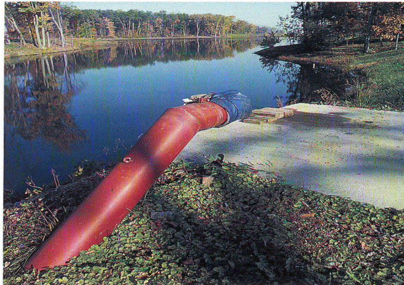
Figure 2 - Details of a dry hydrant installation
